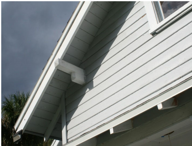
Exposed rafter ends and purlins
